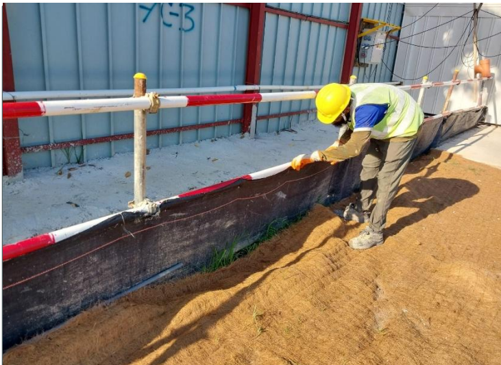
Check silt fence and replace if torn
