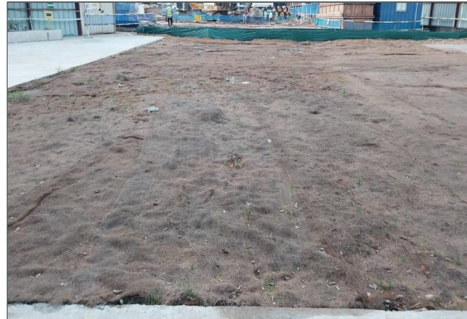
Cover bare earth with erosion control blanket
