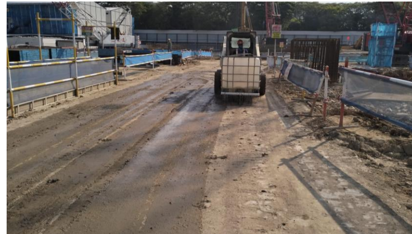
Recycled water used for Daily Dust Control (watering)
