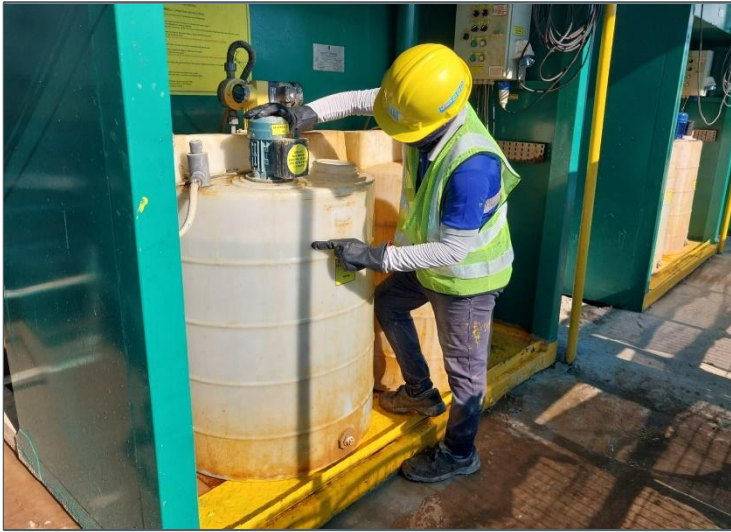
Check ECM treatment plant chemical level
