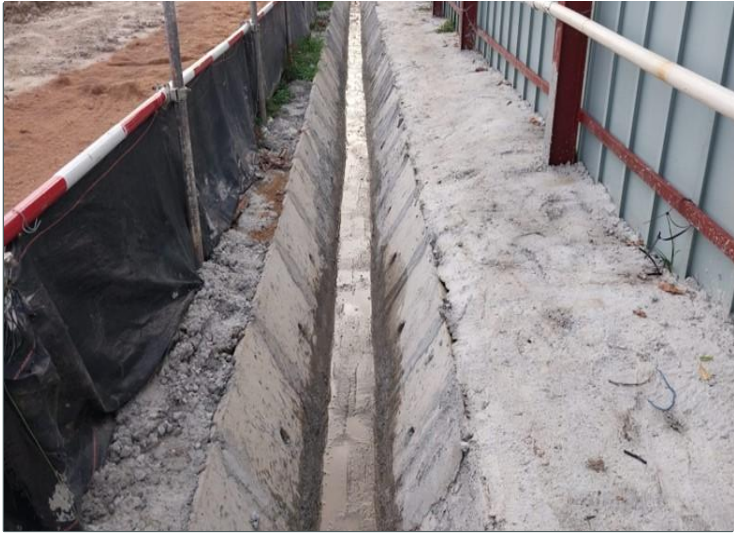
Silt Fence with Cutoff Drain
