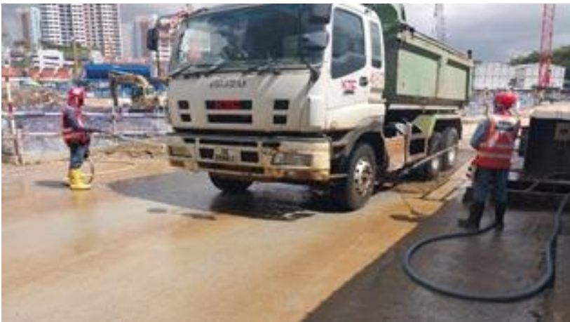
Recycled water used for Washing Vehicles
