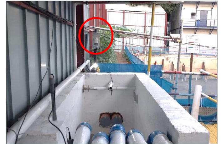
CCTV (SIDS) to monitor discharge SILT IMAGERY DETECTION SYSTEM
