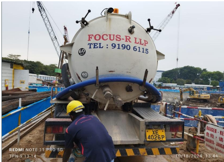
Check and reduce ECM sludge level
